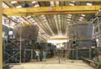
▼ Millmerran - Coal Mills
