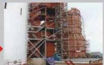
Krabi Power Project Installation of FGD System
