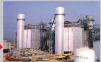
Ratchaburi Combine Cycle Project Installation of HRSC x 2 units
