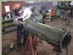
▼ Shuqaiq - Pipe Spool
