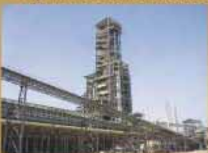
▼ Qatar - DRI Tower Structure
